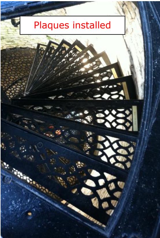
Rear Light steps with plaques installed
