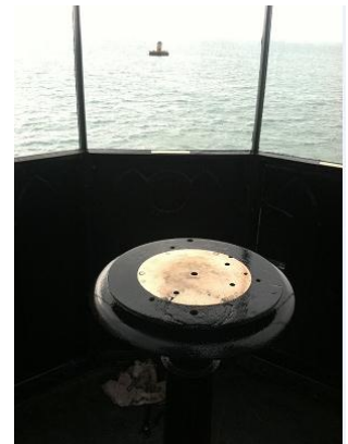
Rescued pedestal from Front Light and installed in Rear
