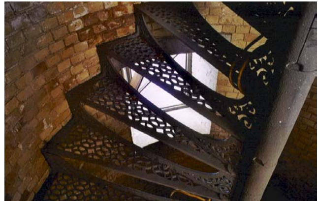
Interior steps before renovation
