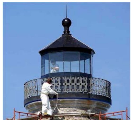
Close up of new decorative railing and ventilator ball
