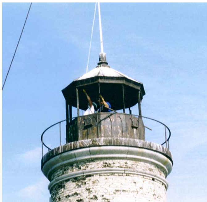
Mihm and Shepard contractors preparing to remove lantern room
